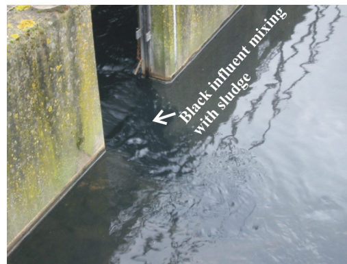
Figure 2.6. Anoxic Zone Mixing.
