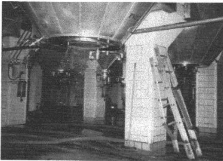
Open fermenter before cleaning; hoses snake across wet floor, ladder rung is loose
