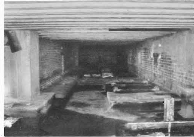
The void beneath Topshop in 2011.
