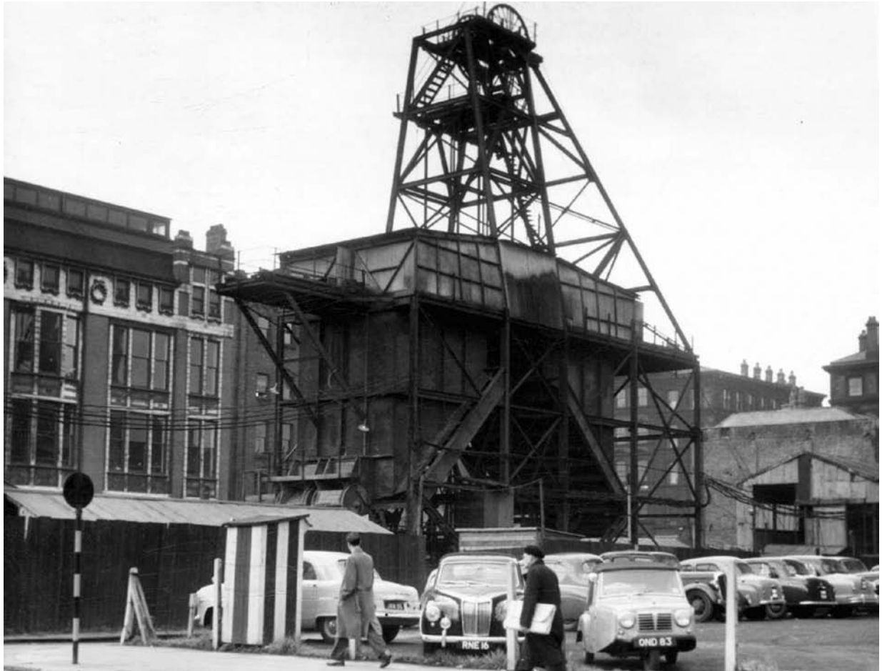
Figure 6. A view, captured in 1955, of the prominent headgear located at Piccadilly needed to winch men and materials to the GUTE tunnel workings. The façade of the exchange at York House, York Street, is to the left of the image. (Source: Photograph by A. Dawson, 1955. Courtesy of Manchester Archives and Local Studies, ref. m56369.)
