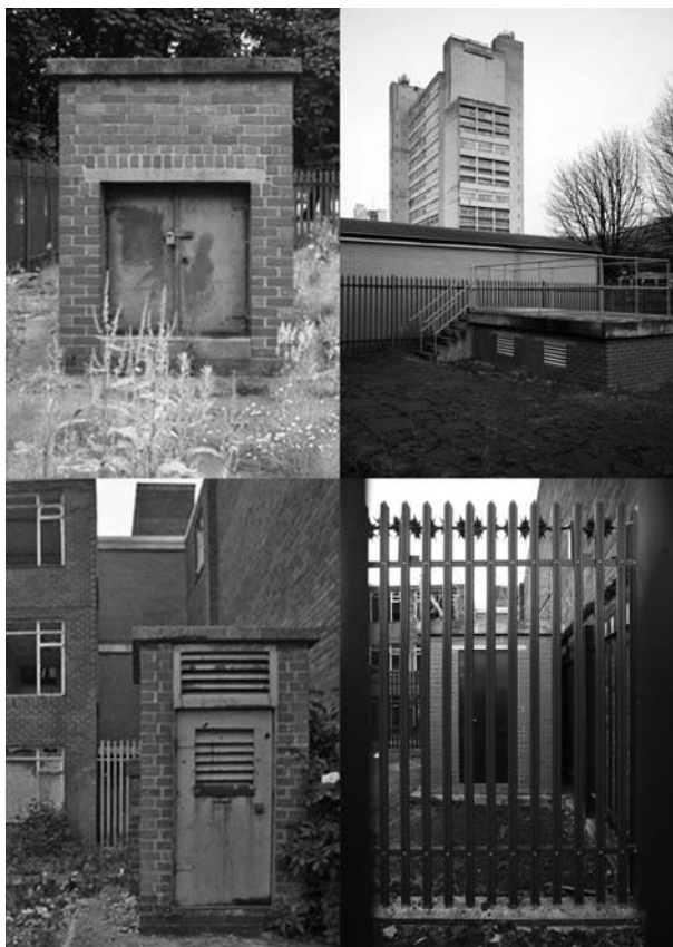
Figure 5. [image top left] The small surface building at the top of cable tunnel as originally constructed, Lockton Close, Ardwick, Manchester (Source: Courtesy of George Coney). [top right] The same location after being rebuilt and secured in 2005 (Source: Richard Brook). [lower left] The small surface building at the top on cable tunnel, Islington Street, Salford (Source: Courtesy of George Coney). [lower right] Additional security fencing installed around Islington Street access point. (Source: Richard Brook).
