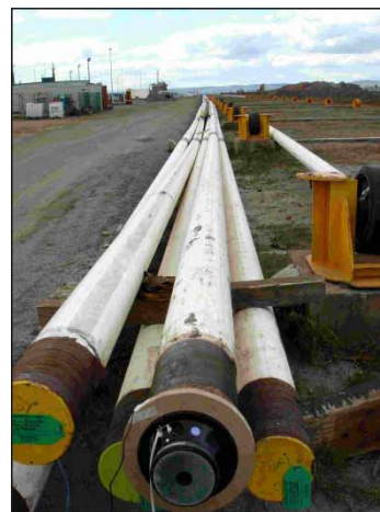
Fig. 6 524 m length of steel pipeline
