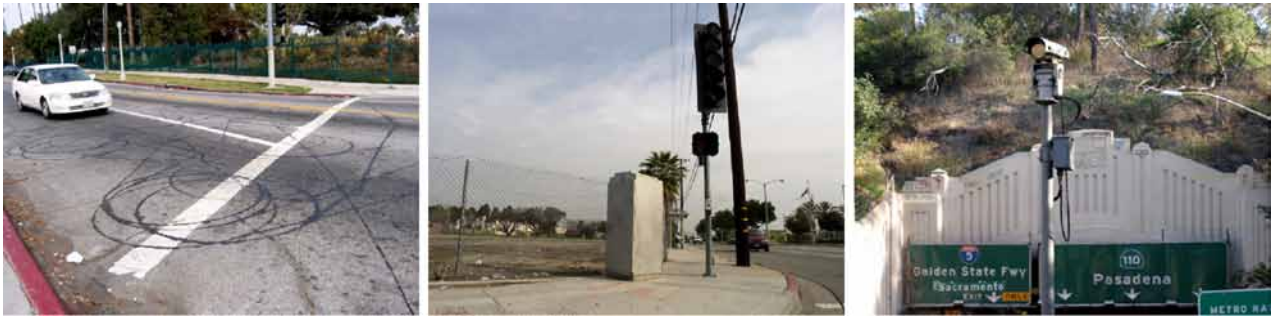
Figure 5. Examples of coded infrastructures enrolled to monitor and control traffic flows in Los Angeles. Picture left: shows black swirls of induction loop under the road's surface that can detect stationary cars at the junction. Picture middle: a bland control box that adapts the phasing of sets of networked traffic lights according to predict flows. Picture right: a steerable video camera with ANPR. (Source: The Center for Landscape for Land Use Interpretation, < www.clui.org/clui_4_1/ondisplay/loop/exhibit/ >.)
