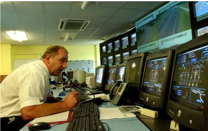
Figure 4. View of a control centre for a road network. The primary interfaces of monitoring and control software are evident on the numerous screens dominating the working space. (Source: Midland Expressway Ltd, < www.m6toll.co.uk >.)
